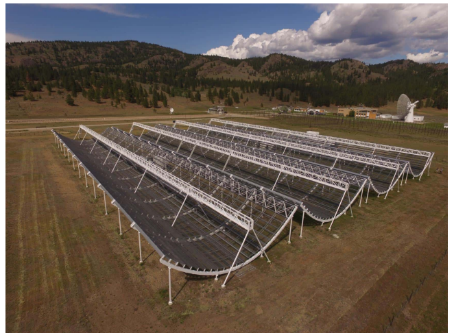
Figure 2: Photograph of the Canadian Hydrogen Intensity Mapping Experiment (CHIME) radio telescope in British Columbia Canada. CHIME is a radio interferometer. Image credit CHIME collaboration.
